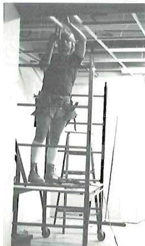
Workmen from State Construction Corporation installing drop ceiling in museum.
